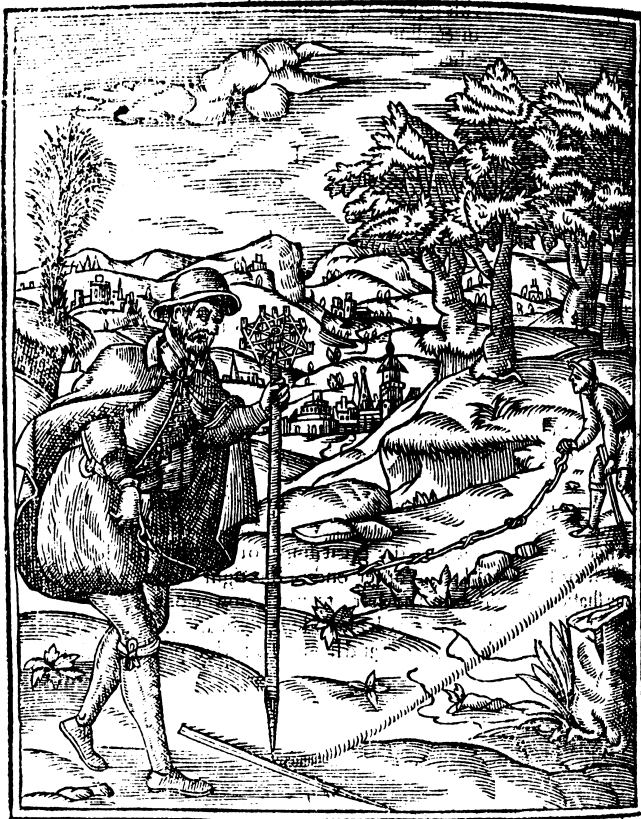
How to reduce all sorts of ground into a square for the better measuring of it.
