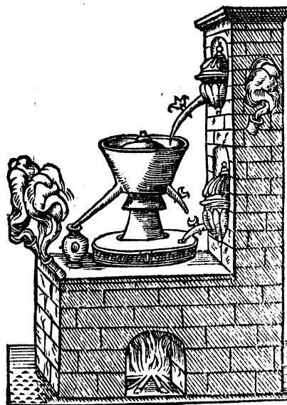
The Venetians distill their water in such an instrument: the furnace is round and containeth on euery side round about it many earthen
